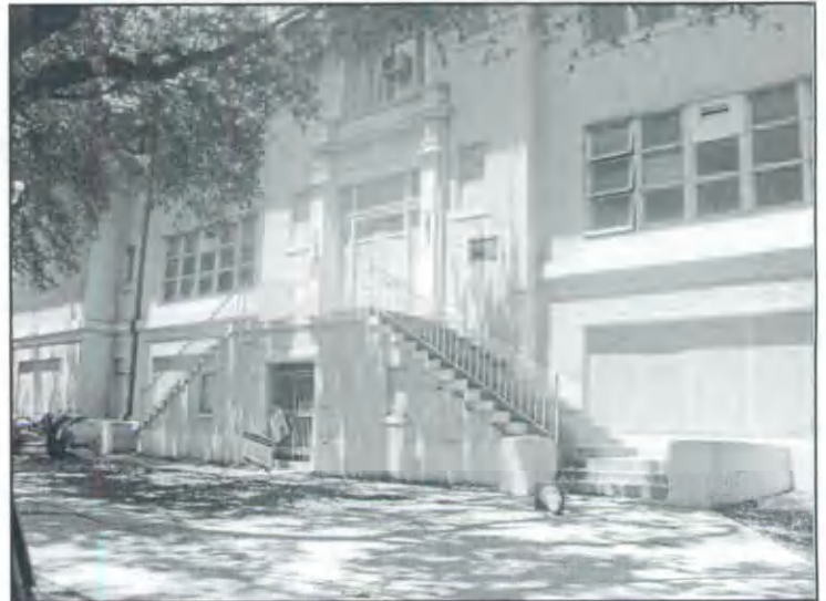
An empty public school in New Orleans, Summer 2006.
