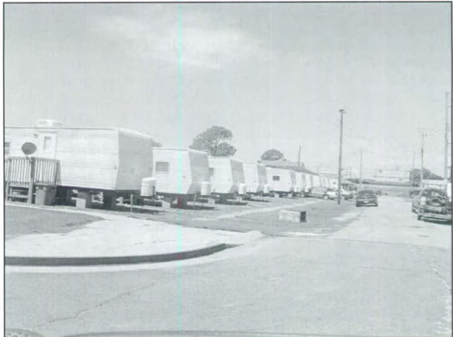
A row of FEMA trailers, 2007.
