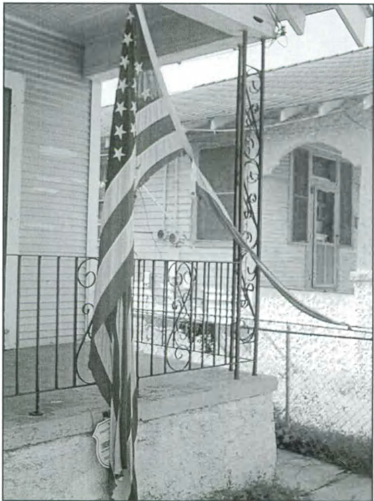
The porch of a destroyed home in the 9th Ward, 2007.
