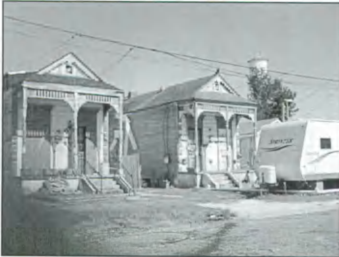
FEMA trailers in front of shotgun houses, 20 months later.
